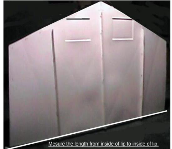
Now you will need to check to see that the lower lip of the end wall is even with the lower lip of the side wall. If the edge of the rear wall is in slightly from the out side edge of the side wall this is ok. You will need to cut the height of the rear wall to fit the roof line and you will need to mark and cut the lips on the inside of the rear wall to fit below the side lip of the roof.
